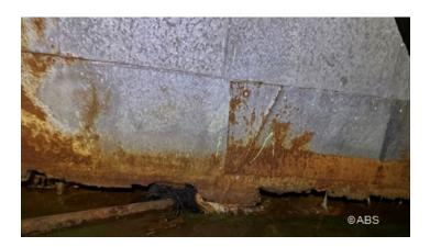
Air conditioning and heating system enclosure wasted
